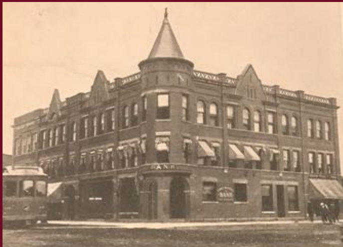
Main office for the Sayre Land and Water Company known as the Lockhart Building located on the corner of Lockhart and Desmond
